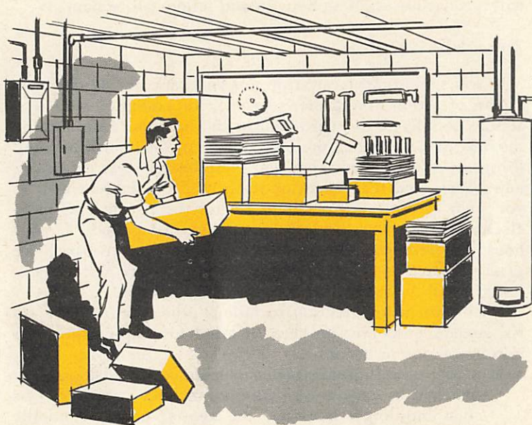
This man is improvising a fallout shelter in a basement corner by stacking heavy material on and at the open sides of a sturdy table. Piling dirt and other heavy material in the basement window wells will improve his margin of protection.
